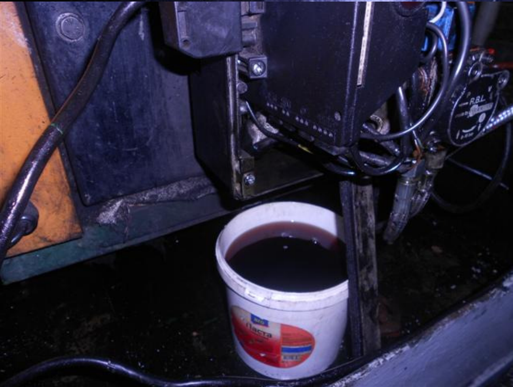
MV Maks: leakage from oil fired boiler, defective switches at boiler and fire pump, missing protection cover, etc
