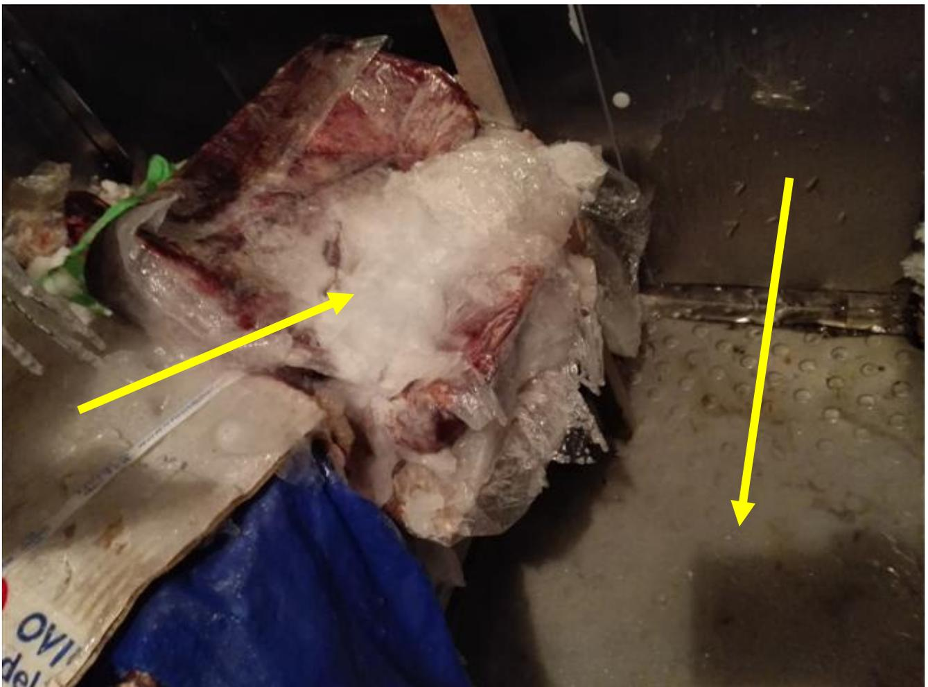
In deep freezer room heavy icing of meat and floor caused by overheating (-10°) and improper gaskets.
