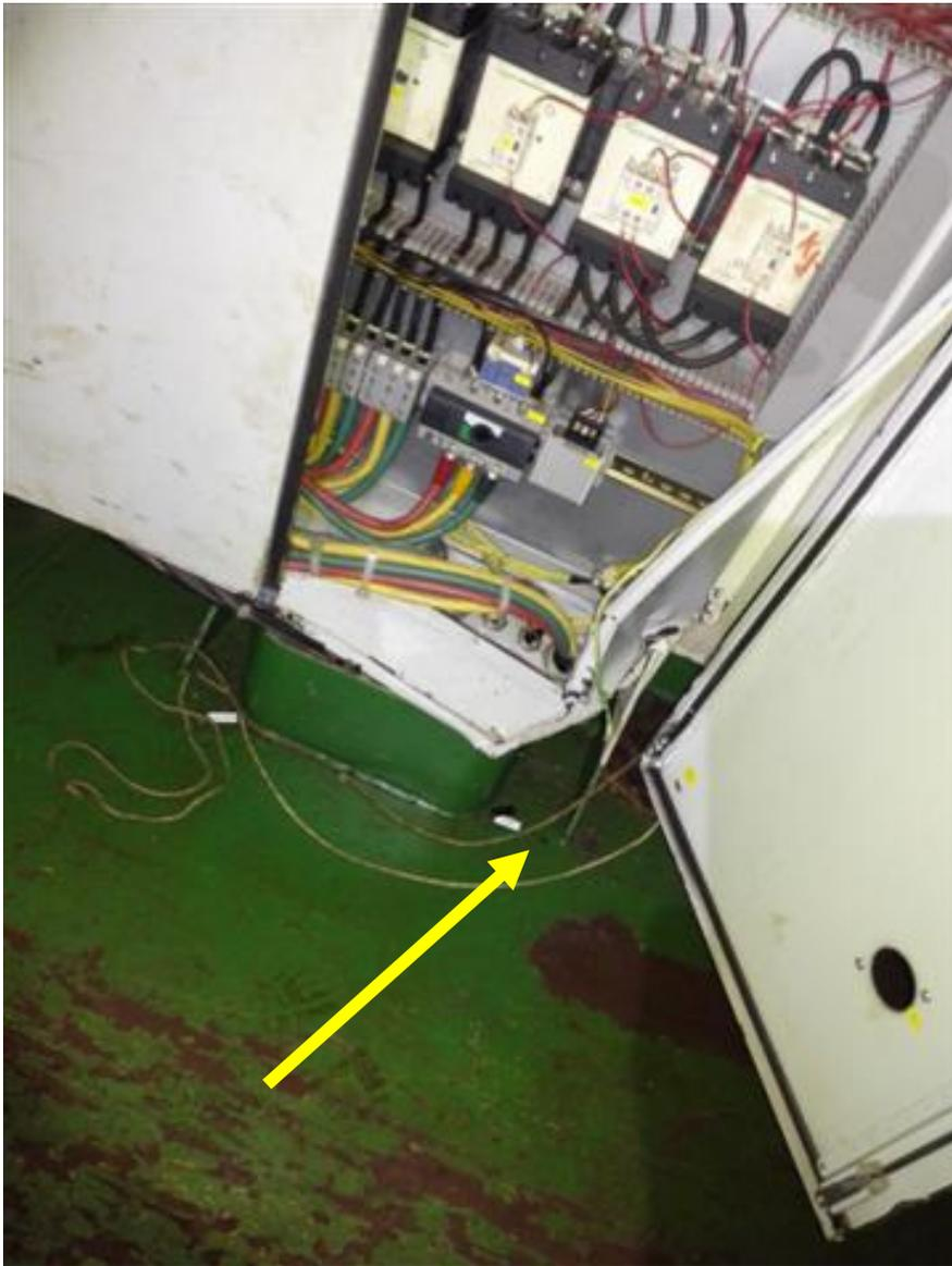
Because of the many unlash drums, both mooring winch control cabinets were heavily damaged. The cabinets were impossible to be closed at all. Crew stated during interview that this had been known for a long time but no spare part orders were forwarded to the company at all. Due to all these facts, this deficiency was recorded with ground for detention.
