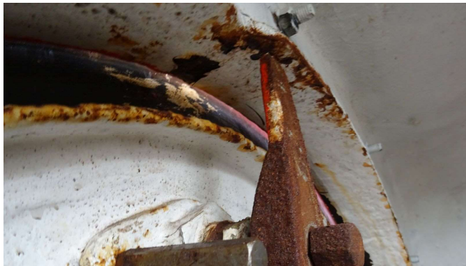
Picture 17 – not closing sash lock
