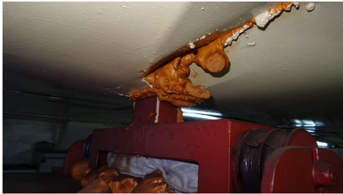
Picture 42 – ceiling in engine control room (ECR)
