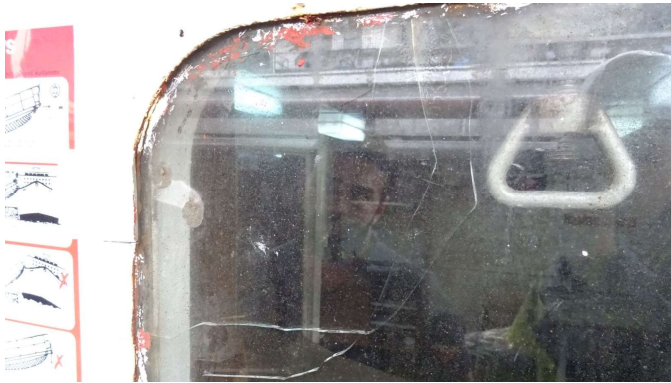
Picture 22 – almost all windows found in...
