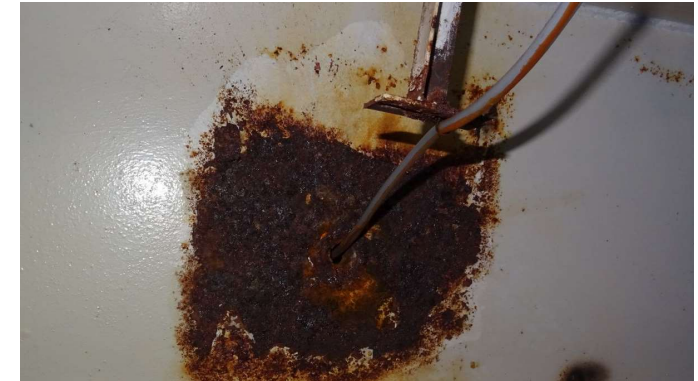
Picture 2 – self-made cable penetrations
