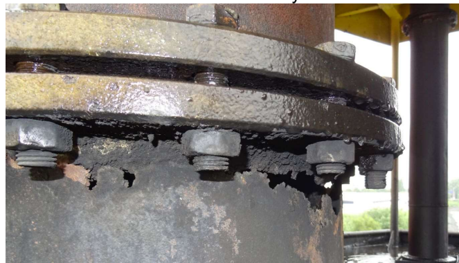
Picture 16 – ...and collapsed due to its own weight
