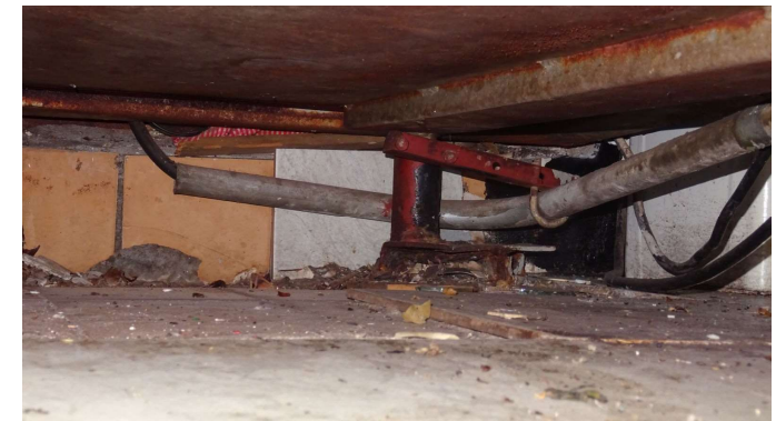
Picture 35 – below the galley cabinets
