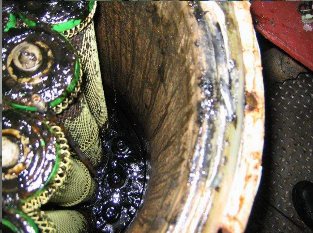
MV Mirvat-I: oil discharged at sea - OWS 15ppm alarm manipulated, filters dirty and not in function, clean water overboard line spoiled with oily residues
