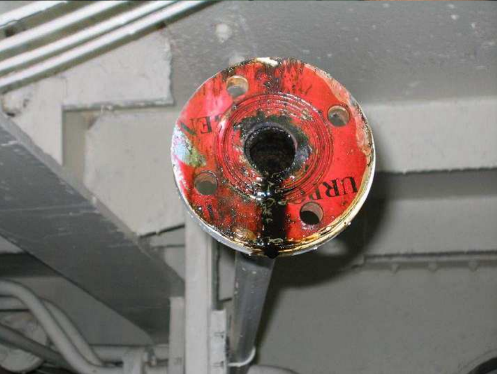
MV Mirvat-I: oil discharged at sea - OWS 15ppm alarm manipulated, filters dirty and not in function, clean water overboard line spoiled with oily residues
