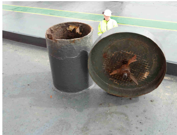
picture 6: and from outside destroyed foundations.
