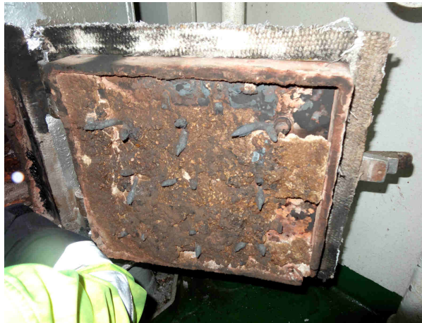
picture 18: damaged incinerator door
