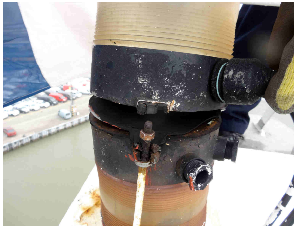
picture 15: navigational lights kept in position by hope
