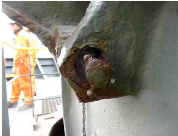
picture 14: bolts and bearings on winches worn out
